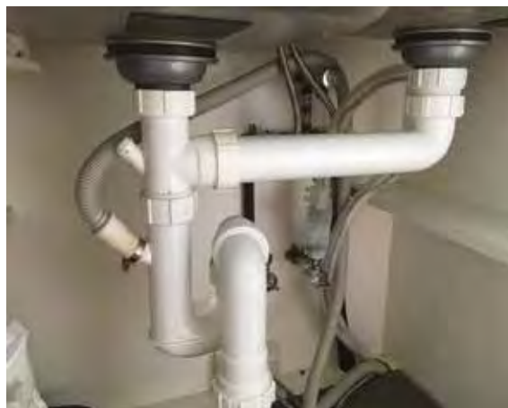
Indicative waste water plumbing and drainage layout
