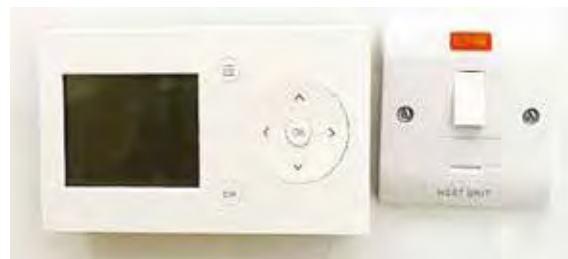
'Indicative central heating electronic programmer
