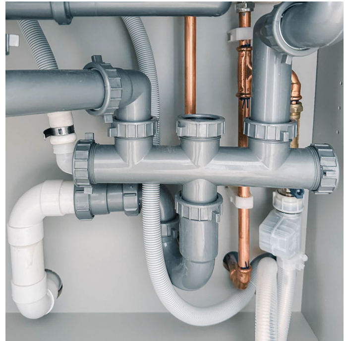
Indicative waste water plumbing and drainage layout
