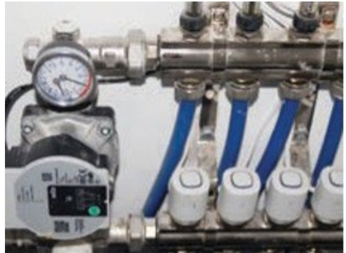
Indicative underfloor heating system
